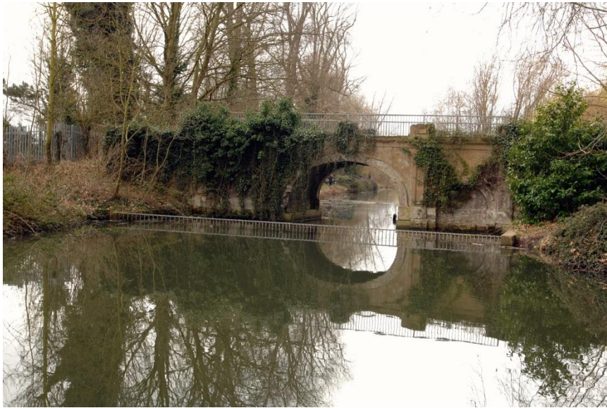
Parklands Bridge before restoration works took place
