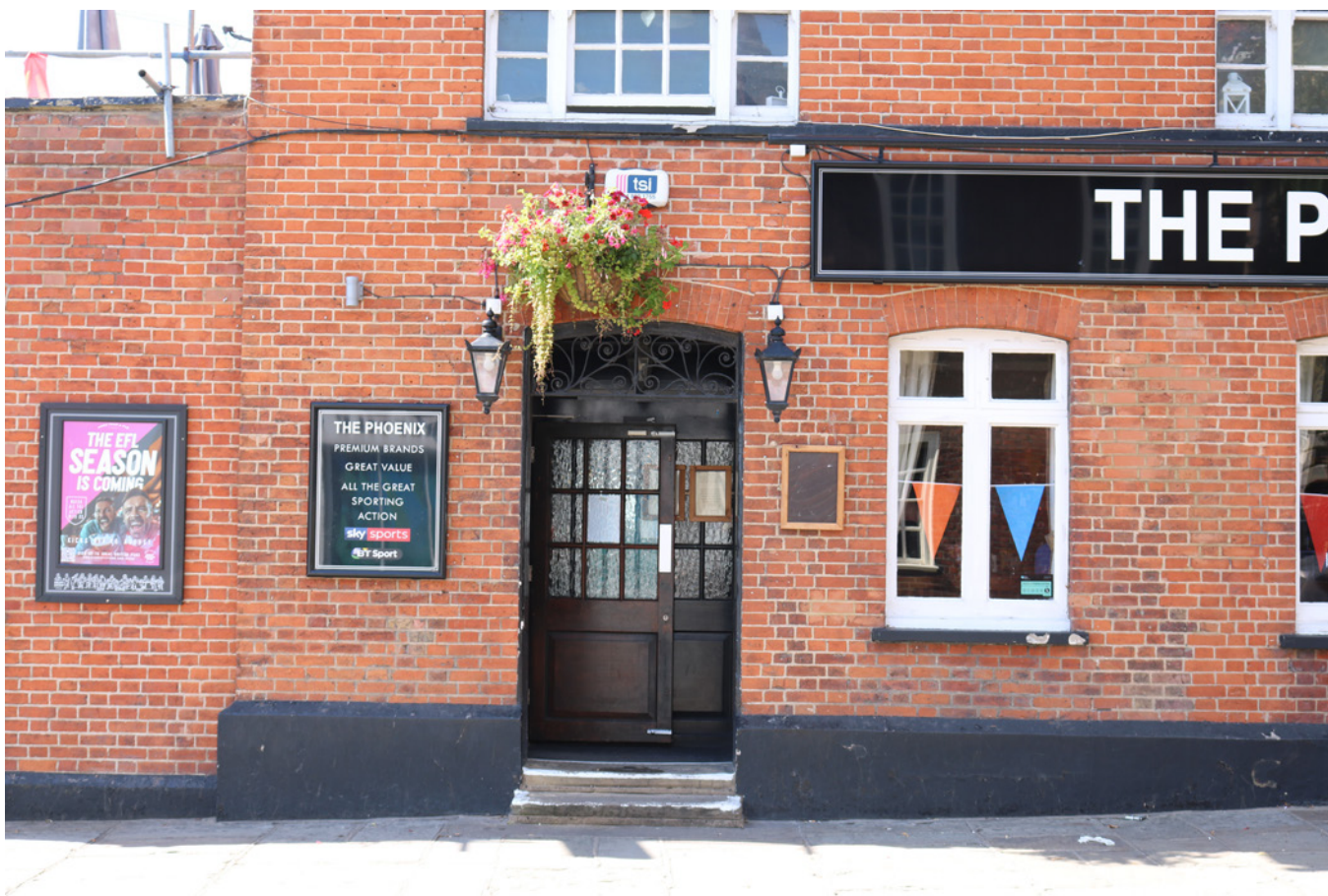
Surface-mounted services & conduit detract from façades
